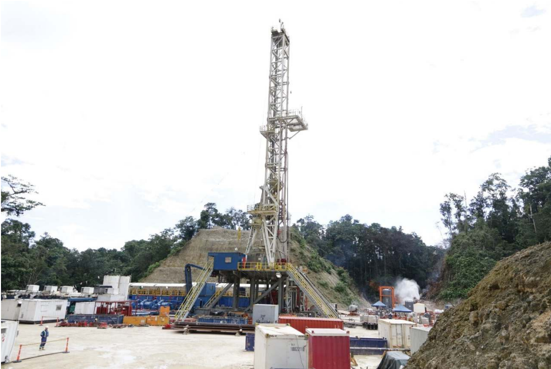
Barikewa 3 well site in Gulf Province.
