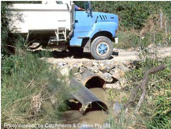
Photo 1 – Temporary culvert formed from recycled steel pipes
