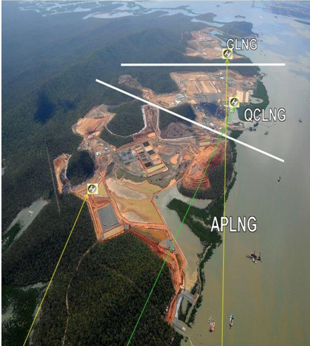
Map 1: Location of Curtis Island LNG Project Sites and their Helicopter Pad Locations
