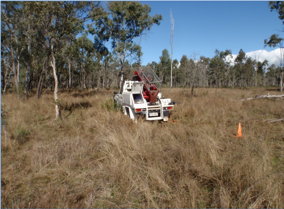
Plate 2: Borehole 23 location, towards the west of the Launch Pad site.
