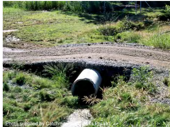
Photo 2 – Temporary crossing of minor drainage channel
