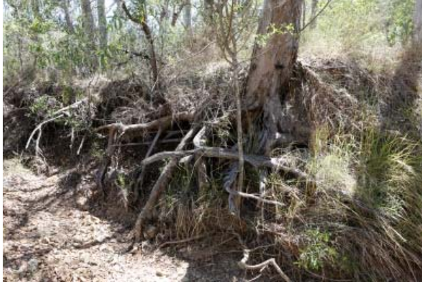
Plate 1 Bank erosion at the KP416.29 watercourse
