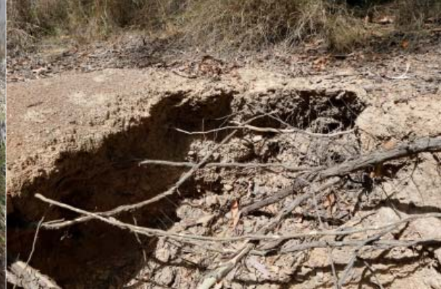
Plate 2 Bank erosion at KP417.72
