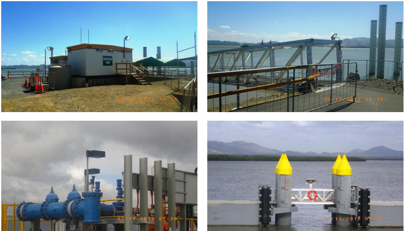
Figure 5: Photographs demonstrating the use of Low Pressure Sodium and Directional Lights with Shrouds to Reduce Light Scatter at the Curtis Island LNG facilities
