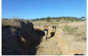
Photo 139 Severe erosion of dam overflow at KP292.45
