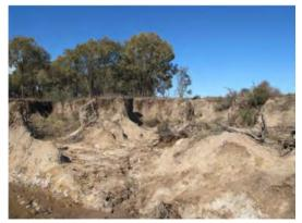
Photo 149 Severe erosion to 4 m in depth at KP307.7
