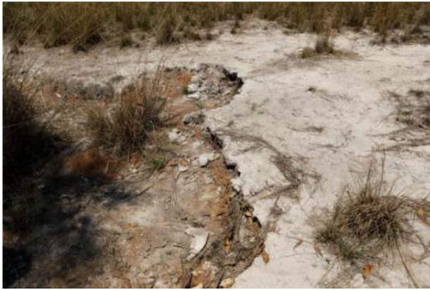
Plate 107 Sheet erosion at KP388.19
