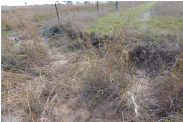
Plate 70 Minor erosion point at KP347.3
